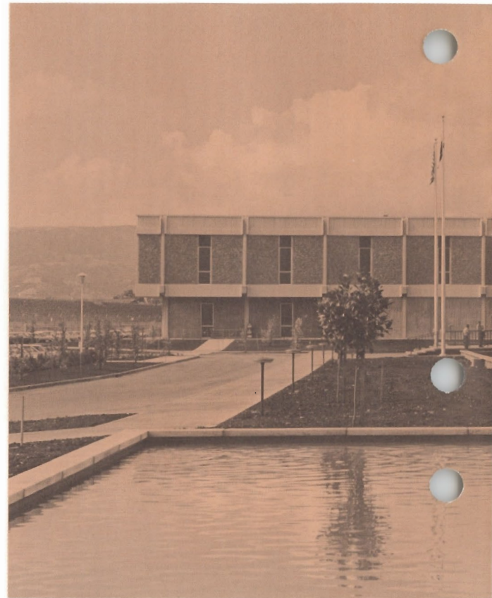
The attractiveness of HP's new Santa Clara facility is obvious in this view across reflecting pool which also serves as secondary supply for emergency fire fighting. The three-building complex includes large roof-top patio, 500-seat cafeteria and 300-seat auditorium. Moving of former F&T Division to Santa Clara freed much needed space for growth by Palo Alto-based divisions.
